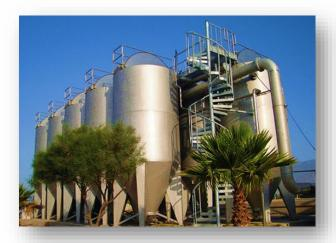
The **DynaLite-Filter** filter employs a backwash rinse that is performed continually while the tank is processing water. An air lift pump, located at the Centre of the module draws the media from the bottom of the filter up into the wash box. As the media is released into the wash box, it falls into the media washer where the filtered solids are separated from the **ZEOSORB**. From there, the filtrate carries the solids out as waste (backwash).
